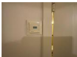
Termostatbryter for varmekabler.
